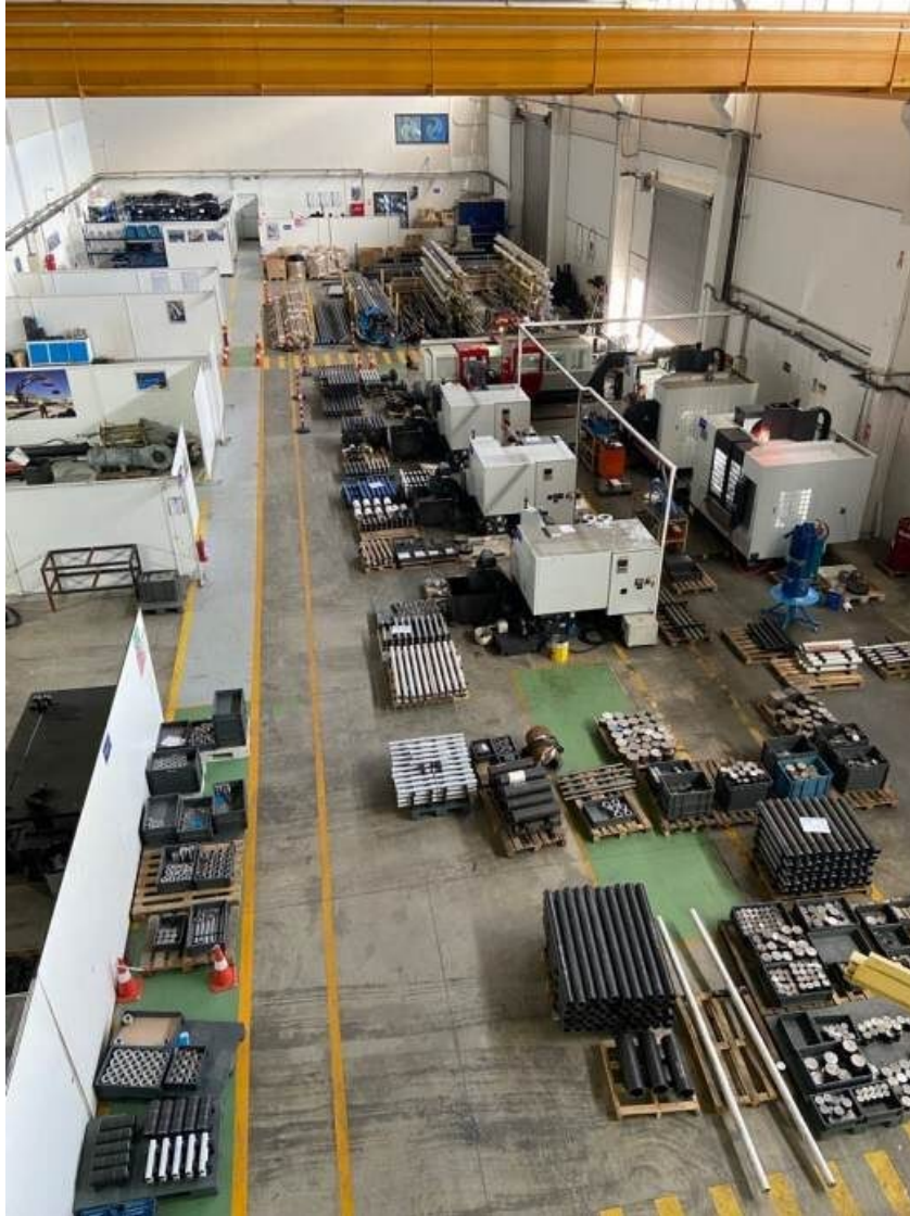
Hydrocyl production floor at AOSB, İzmir: machining, component staging, overhead crane coverage
